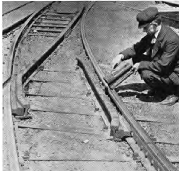
Fig. 3. Cast-Iron Blocks for Guard-Rails, Frogs, etc.*
